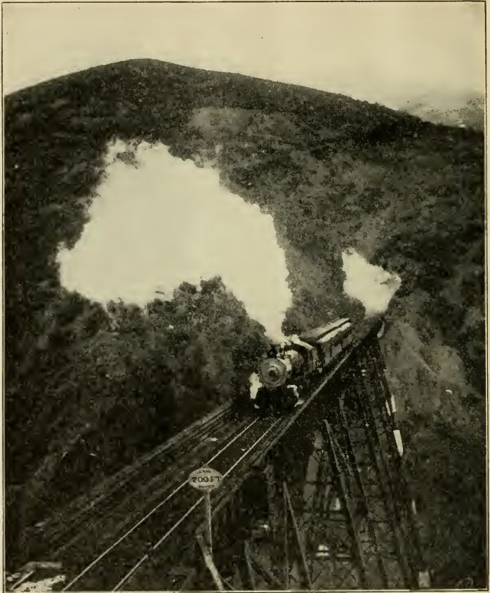
TRESTLE 235 FEET HIGH, BINGHAM AND GARFIELD RAILWAY
